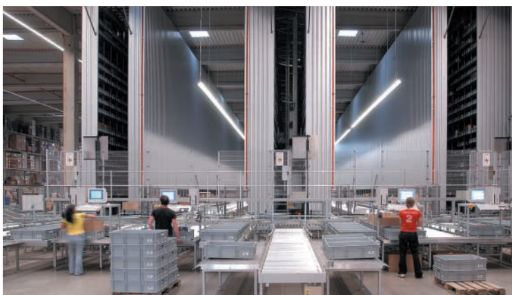
During peak periods, up to five orders can be processed simultaneously at the picking stations of the automatic small parts (mini-load) warehouse
